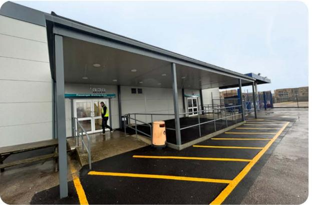
Gradient led the successful delivery of a major refurbishment at Newhaven Ferry Terminal on behalf of Newhaven Port Properties. This £1.8 million project focused on upgrading the terminal's external elevations, including new cladding, windows, doors, canopies, and fire escapes.
